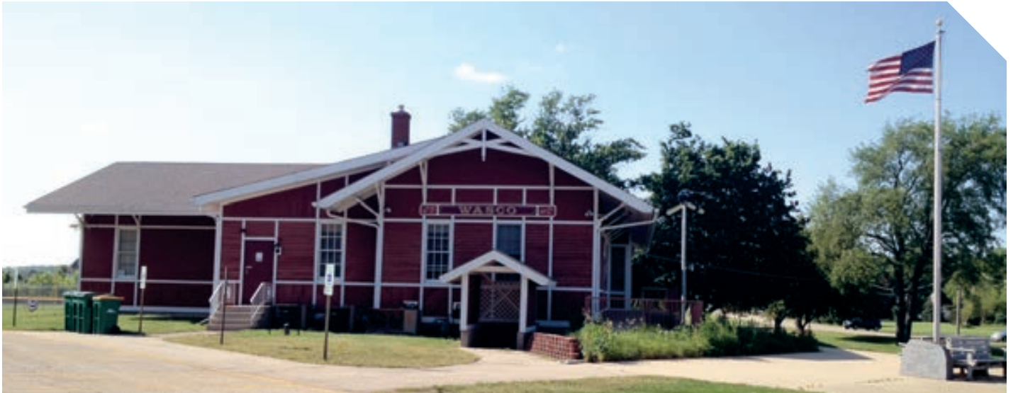
The Campton Hills Community Center.
