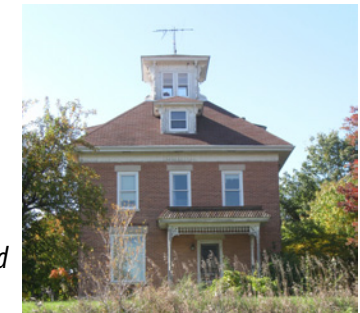
Figure 1.12: Older home along Bolcum Road
