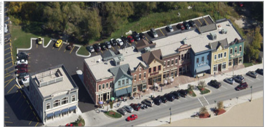
Intermediate walkways allow pedestrians to access various parts of a site, such as walking from a rear parking lot to the storefronts along the main street.
