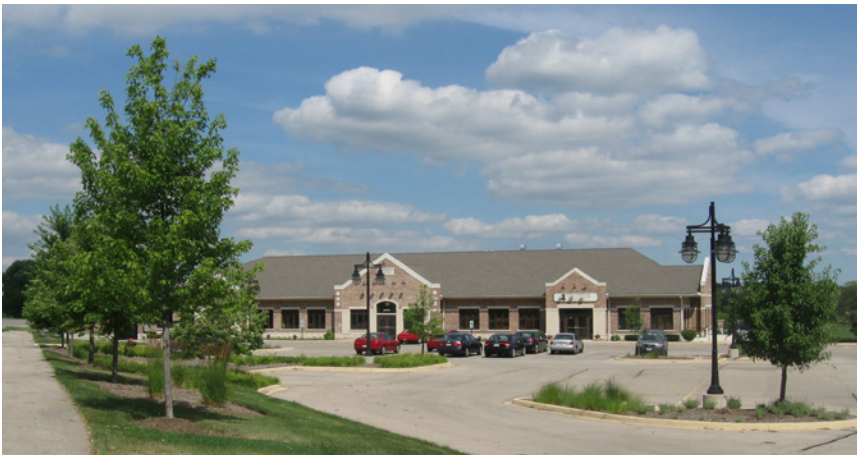
Figure 1.2: Office building constructed along Wasco Road just north of Great Western Trail
