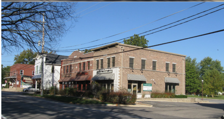
Figure 1.14b: Newer buildings in Wasco
